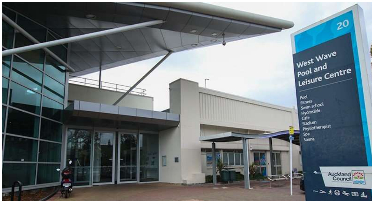
Figure 3: West Wave Pool and Leisure Centre Entrance
